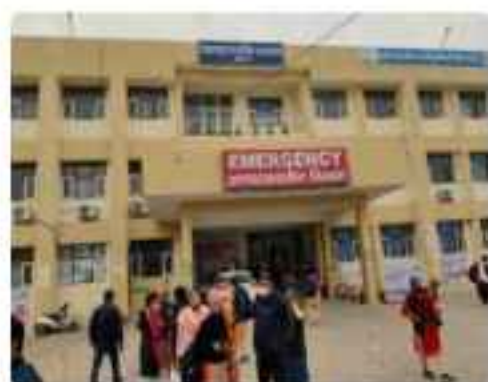
Sub Divisional Hospital, Hodal
